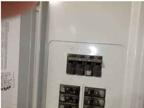
200 amp main for the warehouse section
