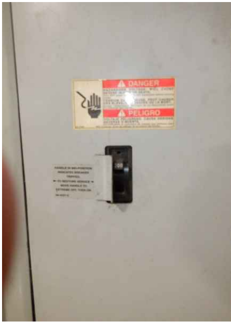
Main breaker feeding the office area panel.
