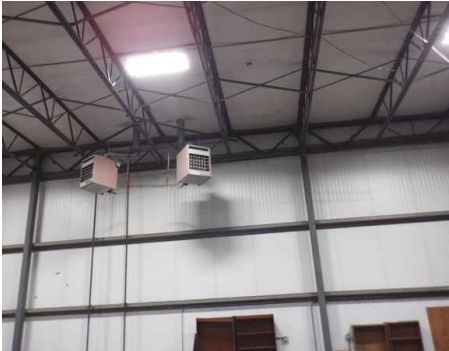
Reznor hanging gas fired heaters on the east side of the warehouse
