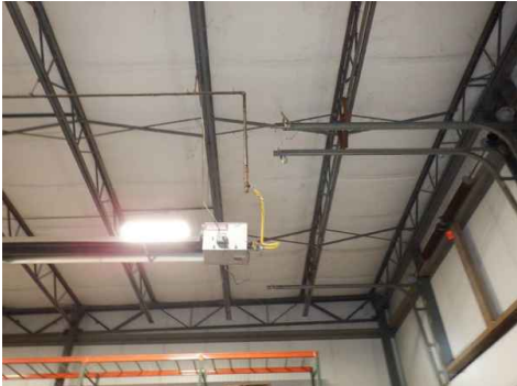
Reznor gas fired tube type radiant heater on the west side of the warehouse.
