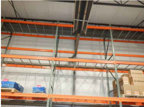
More of the Reznor tube heater
