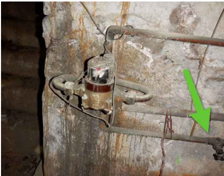
Main water shutoff valve
