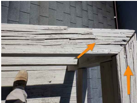
Center stair horse is cracked and in need of replacement.
