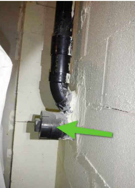
Either valve will shut off the water to the building.
