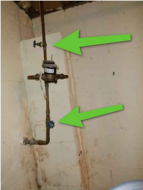
Either valve will shut off the water to the building.
