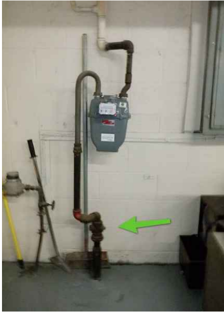
Gas Meter and shutoff valve
