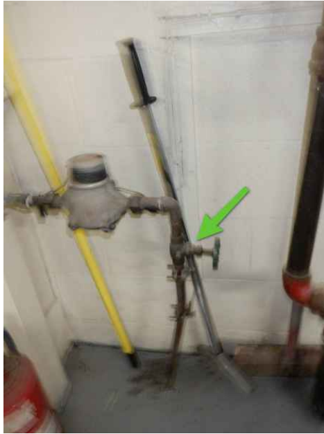
Water Meter and shutoff valve
