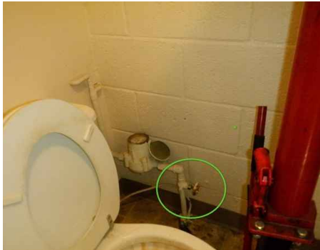
Water Main shutoff valve.
