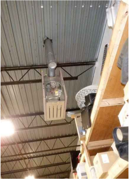
Disconnected heater in the front of the warehouse.
